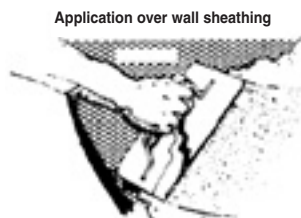
Application over wall sheathing
